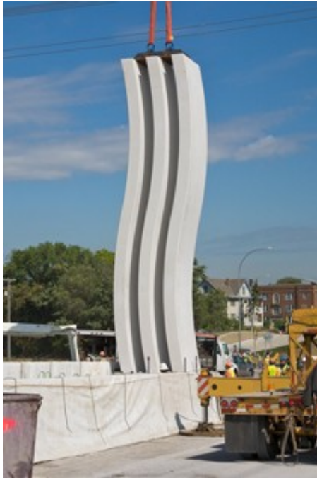
NO x binding (Smog abatement): Minnesota new I-35W bridge sculpture
